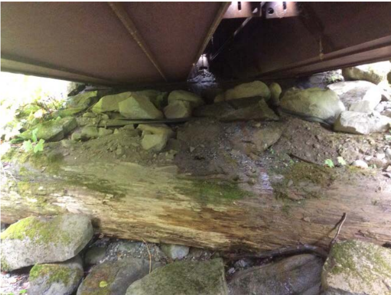
Left Bank Abutment when facing downstream
