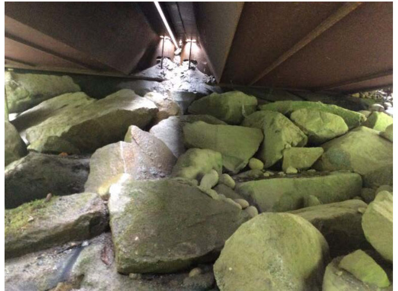
Right Bank Abutment when facing downstream
